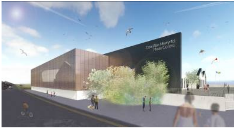
Main façade from Beach Road West
